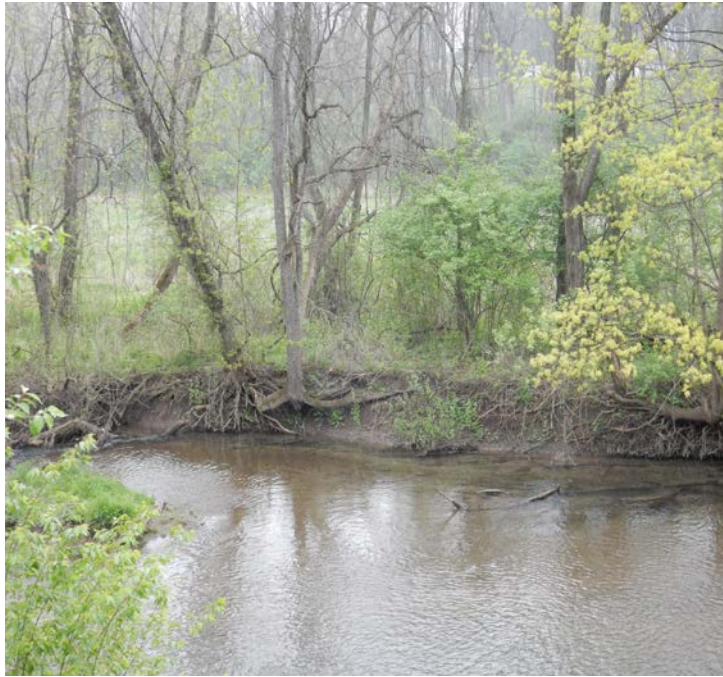
Photograph 1. Eroded section of Spring Creek adjacent to Spring Creek Estates
