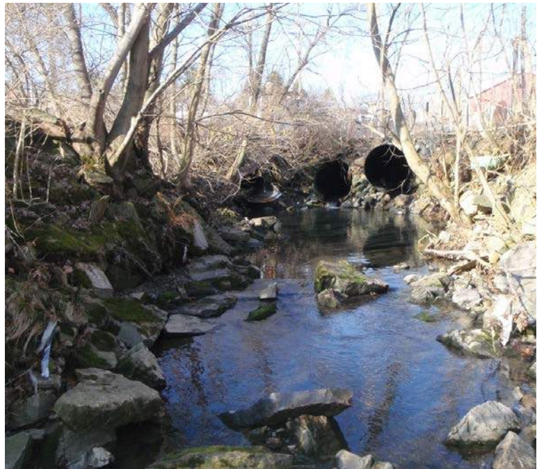
Photograph 3. Stormwater discharge pipes at the beginning of the project reach
