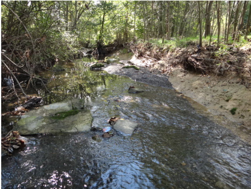
Photo #1 Culvert Inlet
