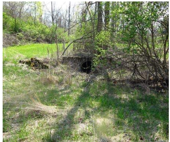
Photograph 2. Outlet structure for Willowbrook Basin (BMP A7)
