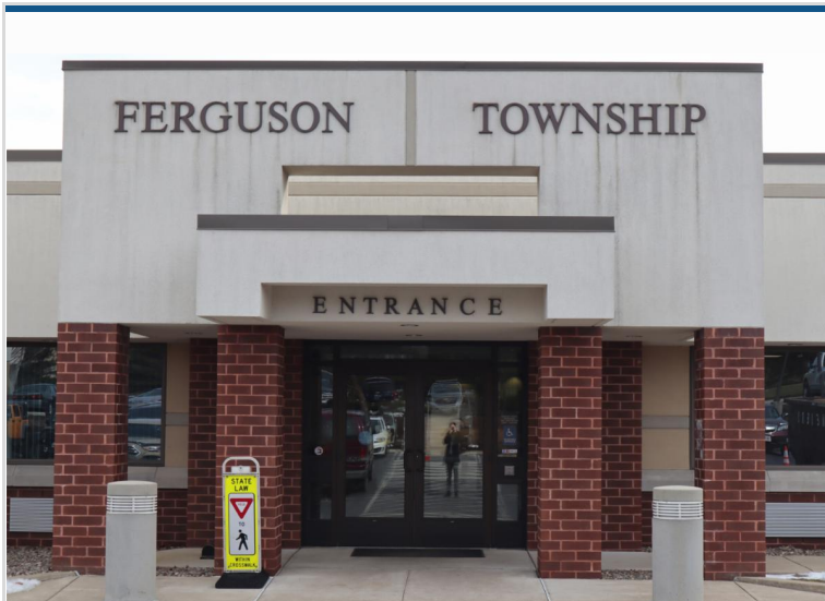
Pictured Above: The Ferguson Township Municipal Building.
