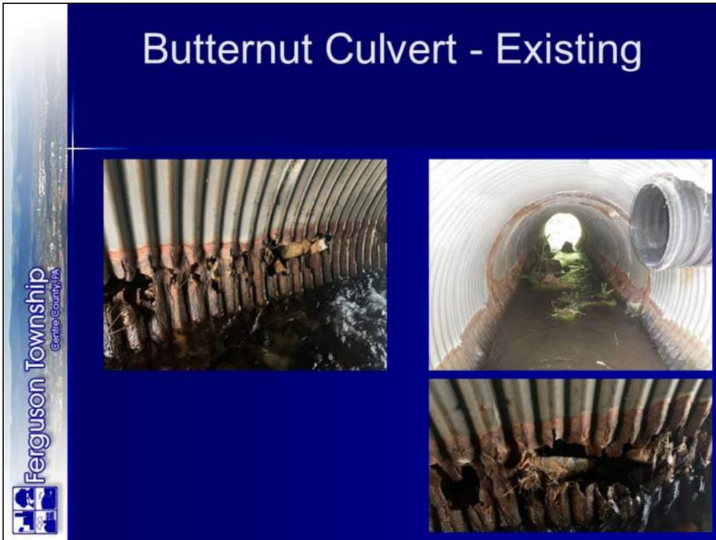
While not part of the PRP, KCI evaluated the Butternut Str. Culvert in July and found the condition Severely corroded
