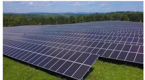
Figure 1 - UAJA's 2.6 MW solar array completed in 2018 was made possible in part by SRE.
