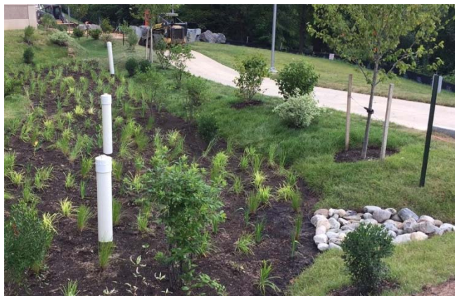
A stormwater structure, such as the bioretention facility above, may qualify a property owner for a credit on the stormwater utility fee.
