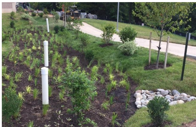
A stormwater structure, such as the bioretention facility above, may qualify a property owner for a credit on the stormwater utility fee.
