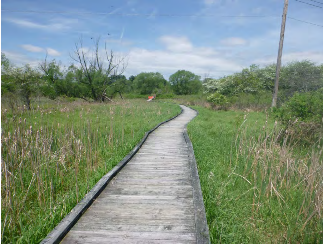
Plate 5.7: View of bridge and boardwalk crossing Thompson Run
