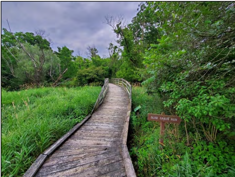
Photo 6 – View northeast of the existing boardwalk bridge over Slab Cabin Run. The sedge meadow to the west (left side of the photo) is dominated by Carex trichocarpa .
