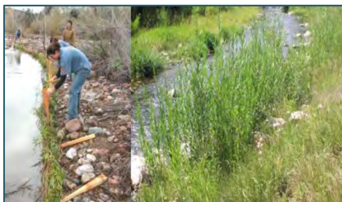
Live fascines during installation (left) and after establishment (right).
