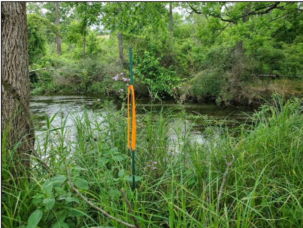
Photo 10 – View west of the proposed new bridge crossing over Slab Cabin Run, in the northern portion of the Survey Area. The existing boardwalk that the bridge will tie into is visible in the right background of the photo.
