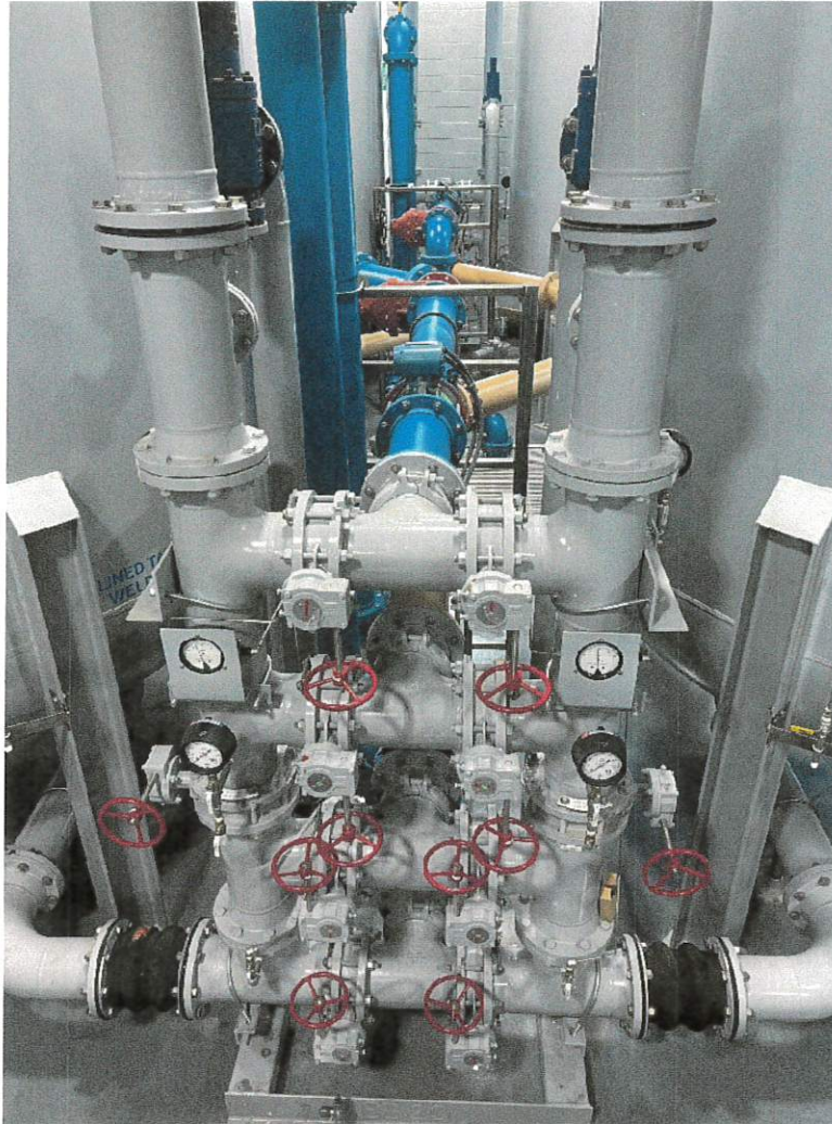
GAC Piping Arrangement
