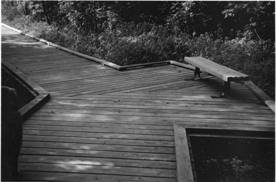
Photo 10A. Example of boardwalk construction for Millbrook Marsh (from Wildwood Lake Sanctuary, Dauphin Co).
