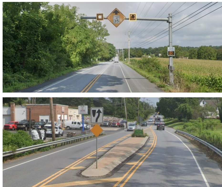
Figure 29. Gateway Traffic Calming on PA Route 41, Chatham, PA
