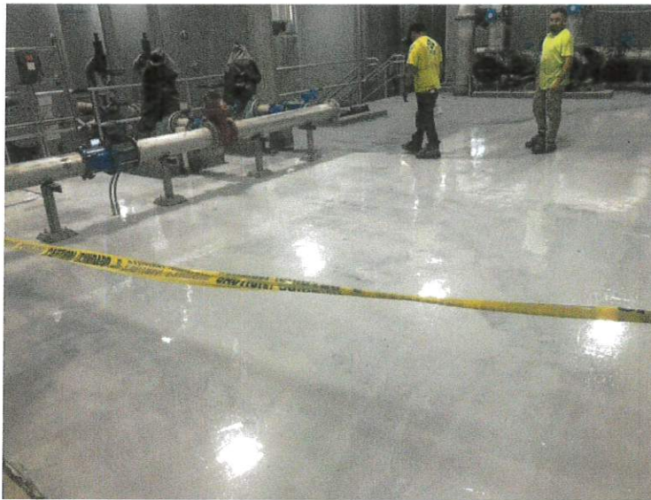
Flooring Installation at UV Units
