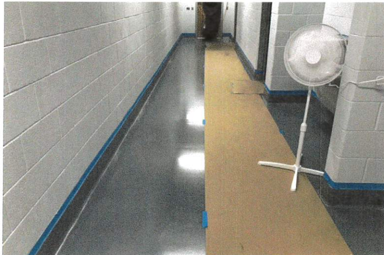
Flooring System in Hallway
