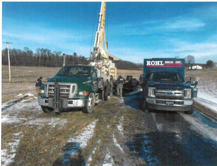
Kocher Well Installation
