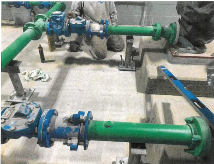
Membrane Filtration Recycle Pump Installation
