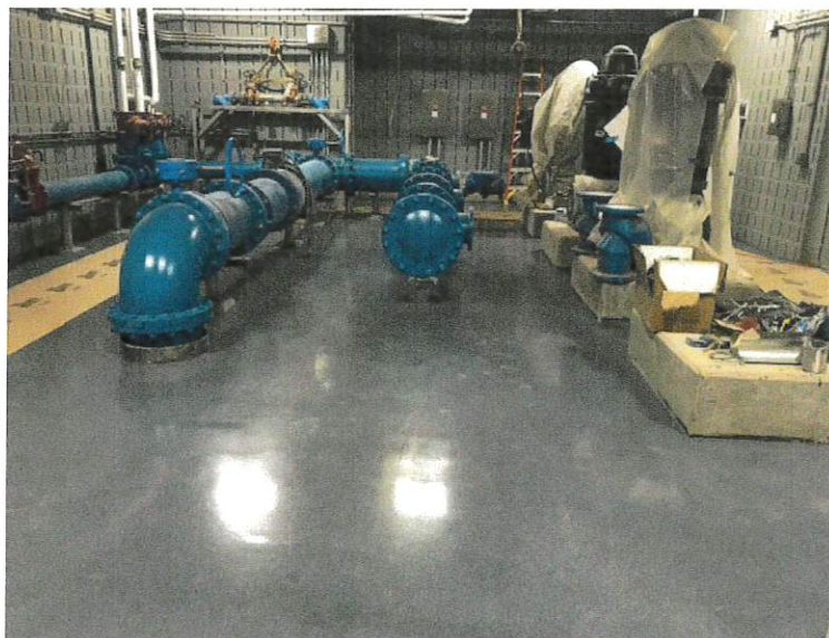
Finished Water Pump Pipe Painting and Flooring System
