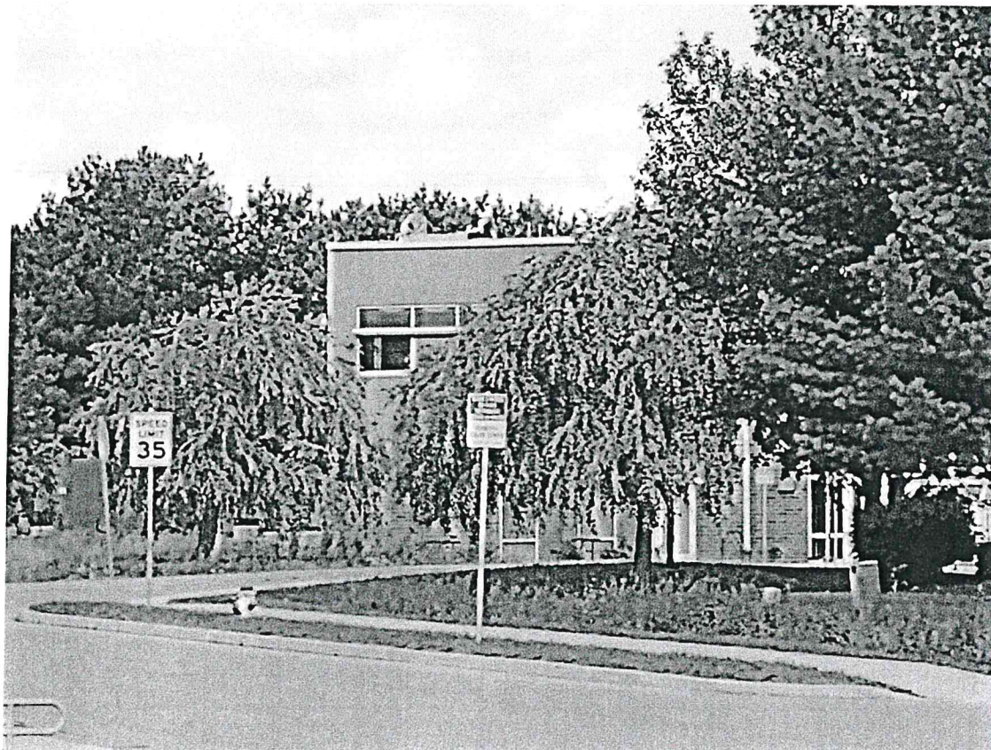
Photograph of impact – The cardboard height demonstrates the height of the panels proposed.
