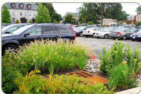
Example of a green infrastructure project to filter storm water runoff from parking areas.
