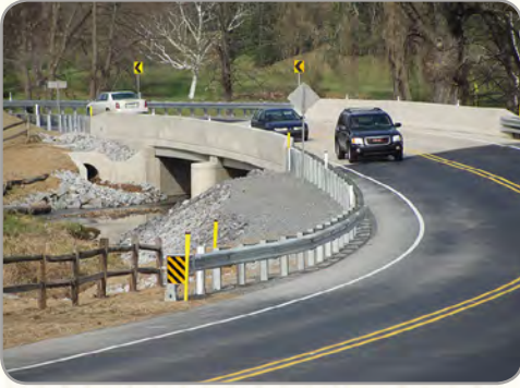
The State Route 3011 Branch Road Bridge was replaced in 2012. The rehabilitation and replacement of structurally-deficient bridges is a primary focus of state and local officials.
