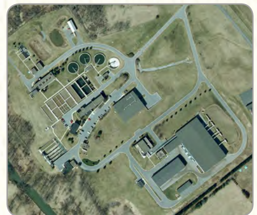
Aerial view of the University Area Joint Authority's Spring Creek Pollution Control Facility.
