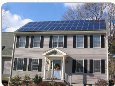
Solar roof panels help reduce energy costs and improve affordability
