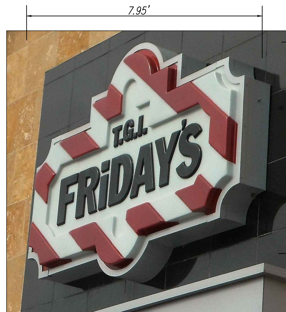
EXISTING SIGN 'H' NOT TO SCALE T.G.I. FRIDAY'S WALL SIGN 5.50' HEIGHT 43.73 SF MATERIAL: PLASTIC/METAL
