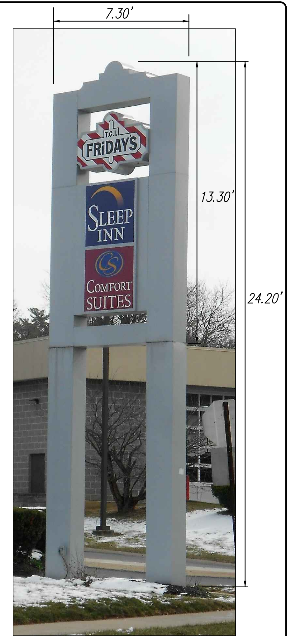
EXISTING SIGN 'E' NOT TO SCALE GROUND POLE SIGNS 24.20' HEIGHT MATERIAL: PLASTIC/METAL
