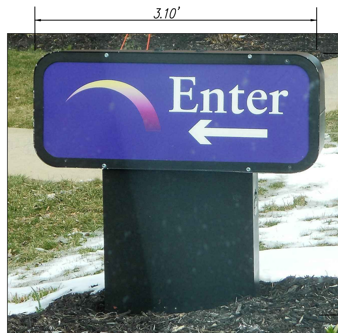
EXISTING SIGN 'G' NOT TO SCALE DIRECTIONAL SIGN 3.05' HEIGHT 3.88 SF MATERIAL: PLASTIC/METAL
