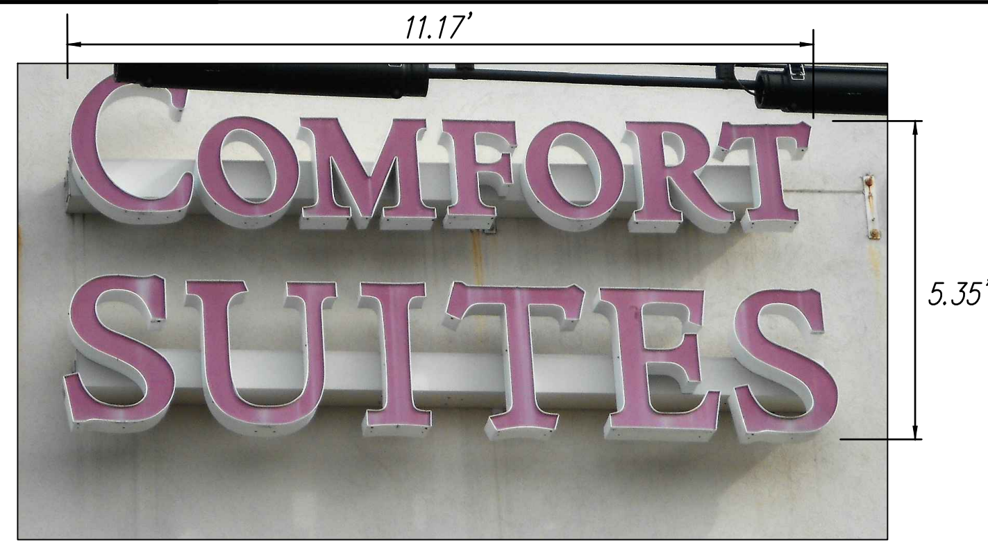
EXISTING SIGN 'C' NOT TO SCALE COMFORT SUITES WALL SIGN 5.35' HEIGHT 59.76 SF MATERIAL: PLASTIC/METAL
