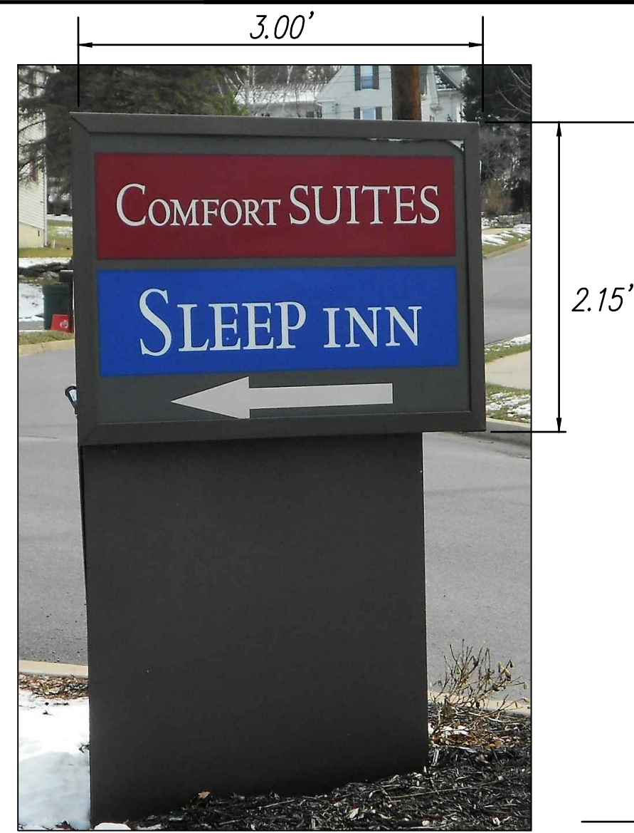
EXISTING SIGN 'B' NOT TO SCALE DIRECTIONAL SIGN 4.70' HEIGHT 6.45 SF MATERIAL: PLASTIC/METAL
